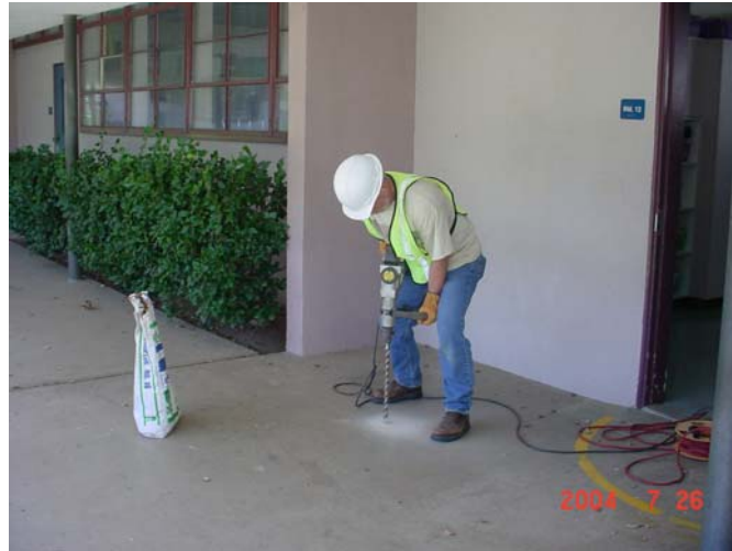
Photo 3 – Drilling hole through slab (1/2" OD).
